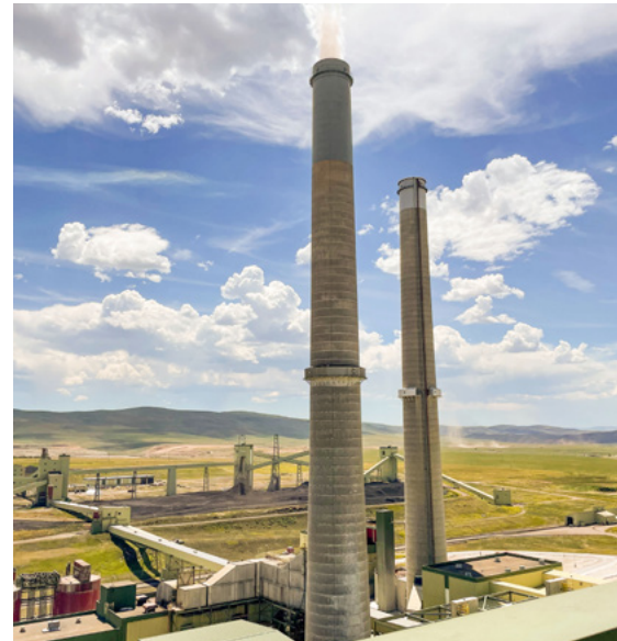
Students toured the Craig Station Power Station during camp.
