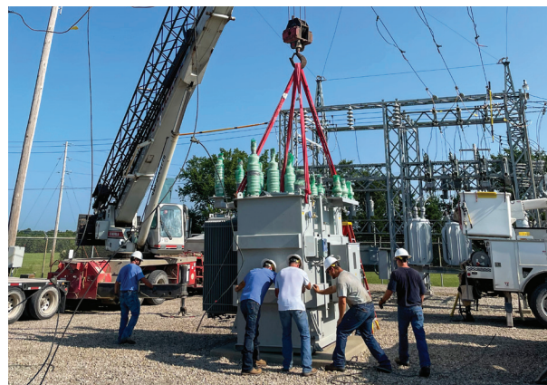
The 4 Rivers line crew assists with the installation of a new transformer at the Westphalia substation.
